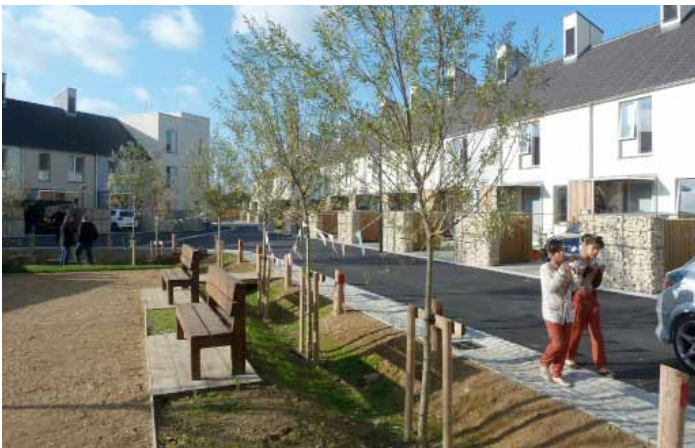
Porous parking reduces water flows to street, dished channel connect site visually and hydraulically and issues to bioswale with a temporary holding capacity of just over 50m 3 , willows in base of swale transpire water and giver summer cooling + biodiversity benefits. Wet meadow vegetation in swale will filter/clean water before it is sotred some more in storm crates. Overall the capacity of the to hold ontl water is greatly increased.
