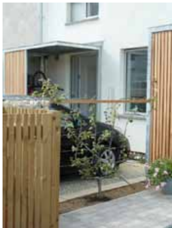
Porous paved parking allows moisture to percolate espalier apple fences - water & food connected
